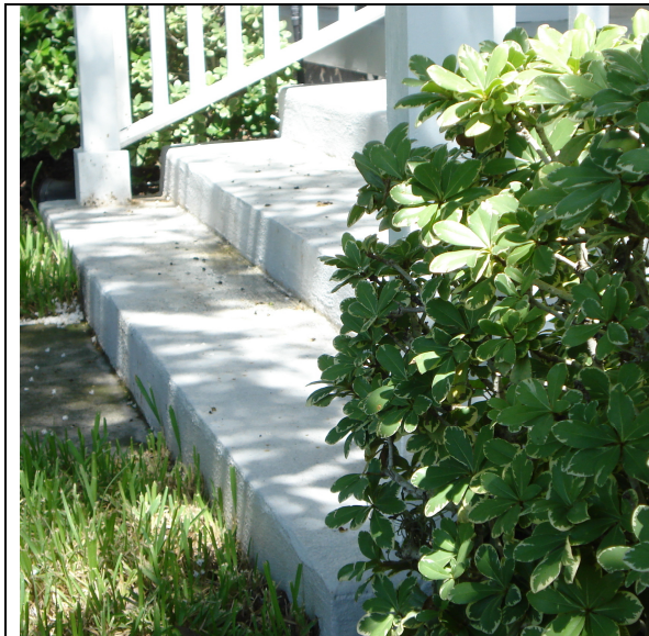
Pavers may be installed on steps with straight edges; bull-nose pavers are required
