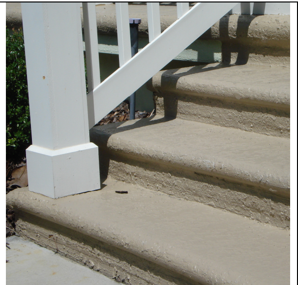
Pavers may not be installed on steps with round edges
